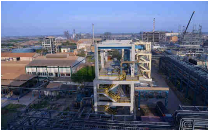
Hydrochloric Acid Plant
