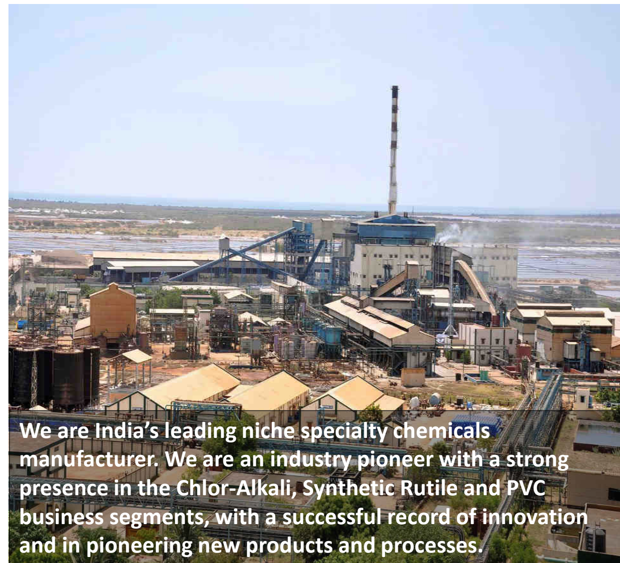
Aerial view of Sahupuram facility
