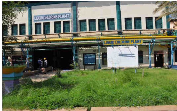
Liquid Chlorine Plant
