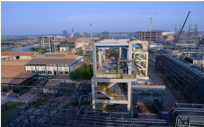
Hydrochloric Acid Plant
