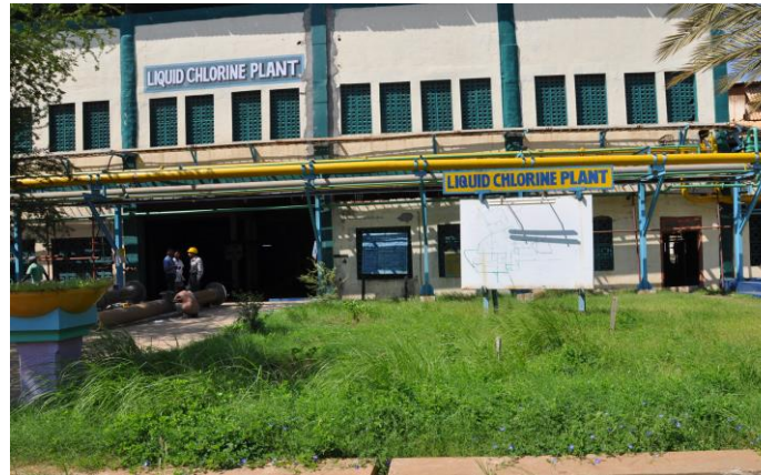
Liquid Chlorine Plant
