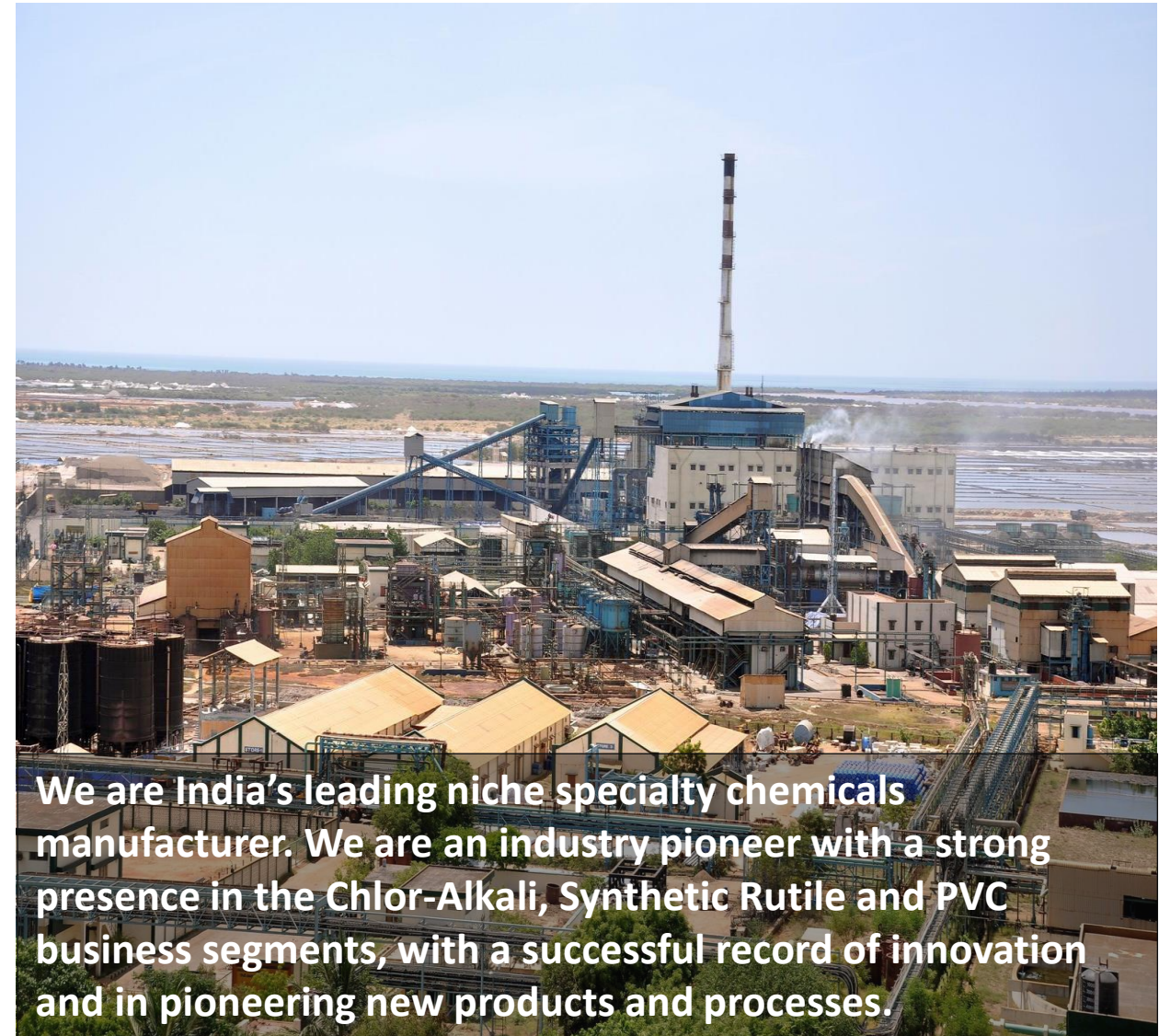
Aerial view of Sahupuram facility
